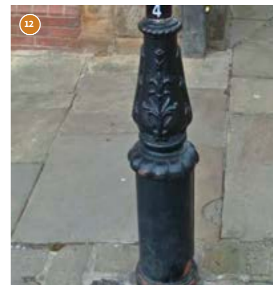
12 TRADITIONAL DETAILING TO BASE OF SOME COLUMNS
