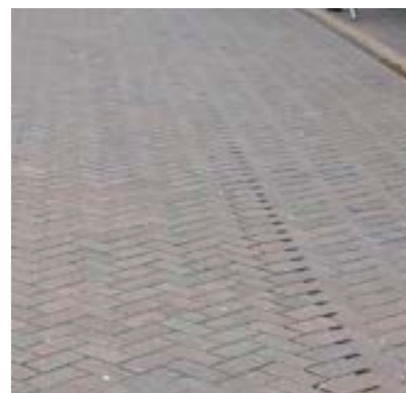
N HERRINGBONE CONCRETE PAVERS ON BURLINGTON STREET
