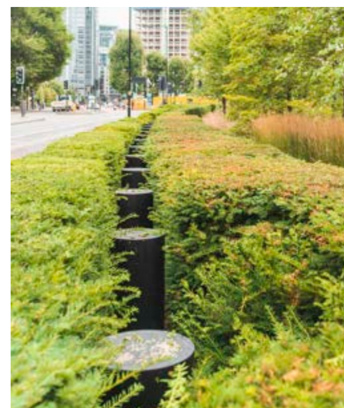
BOLLARDS CONCEALED IN HEDGING
