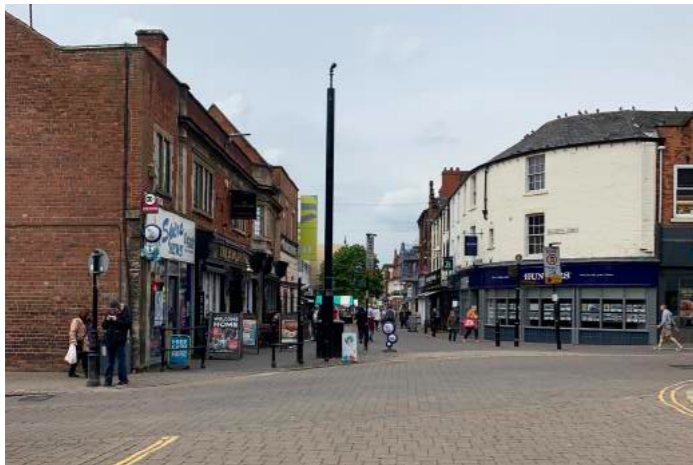
CCTV INFRASTRUCTURE IN RYKNELD SQUARE
