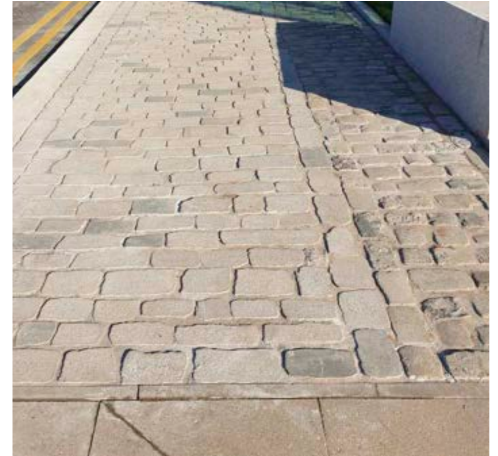
SAWN SETTS RE-LAID NEXT TO UNTREATED COBBLES IN LIVERPOOL; OPTION TWO
