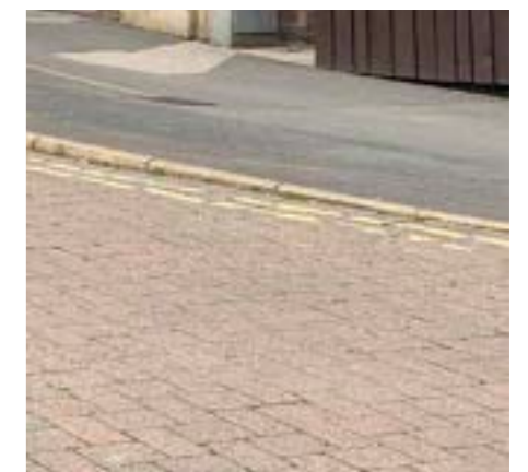
HERRINGBONE CONCRETE PAVERS AND TAR-MAC ON CORPORATION STREET
