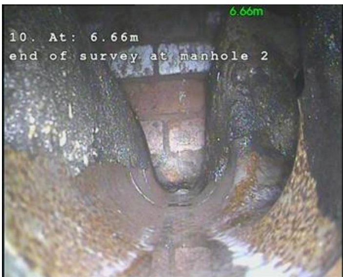
10. 6.66m End of survey at MH2
