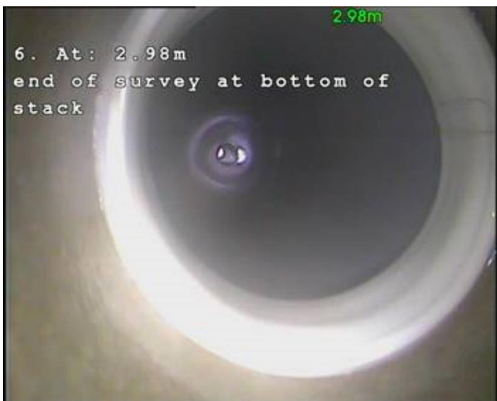
6. 2.98m End of survey at bottom of stack.
