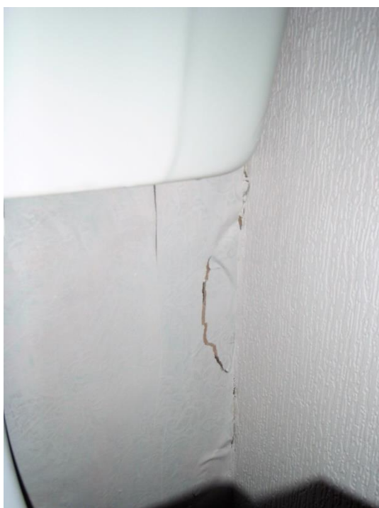
DIAGONAL CRACK BELOW BATHROOM WINDOW BEHIND WC
