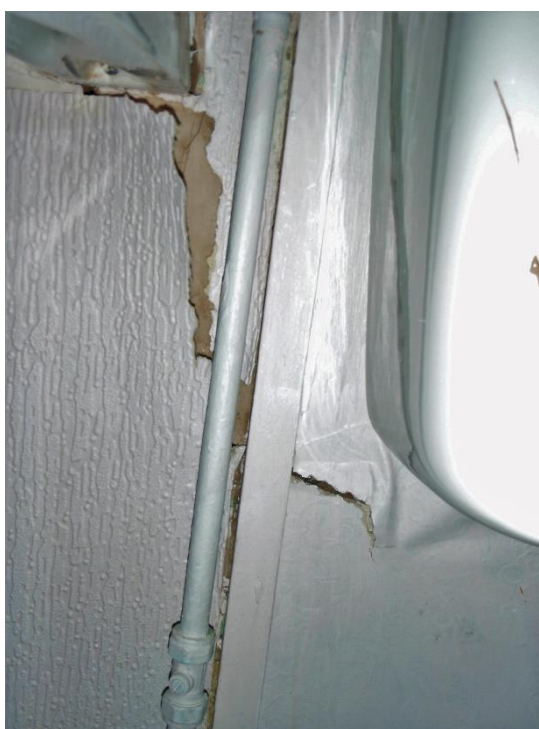
DIAGONAL CRACK BELOW BATHROOM WINDOW BEHIND WC
