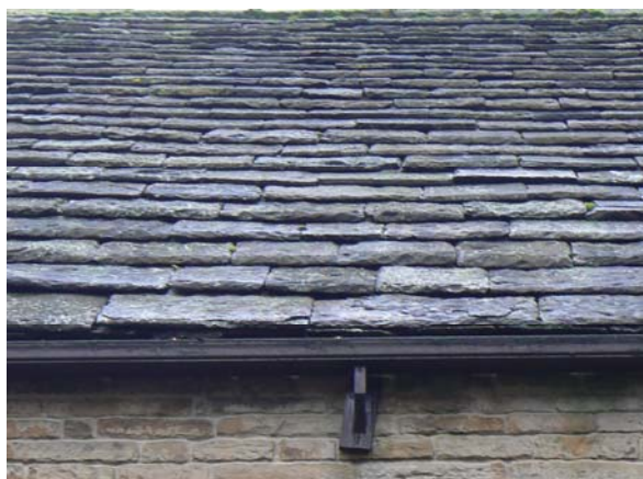
Stone slate roof with timber gutters
