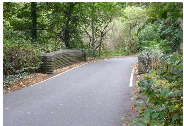
The south bridge over River Hipper
