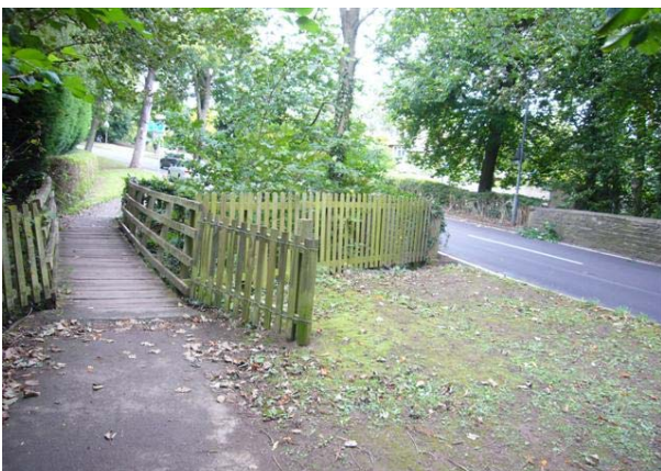
The north bridge and its pedestrian bridge
