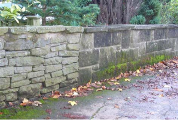
Part of stone wall replaced with cement blocks
