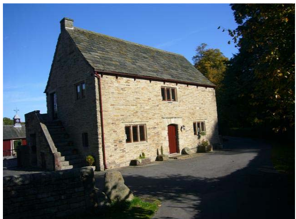
The Stables building
