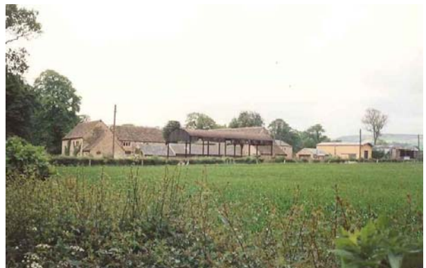
Views of Somersall Hall buildings from north
