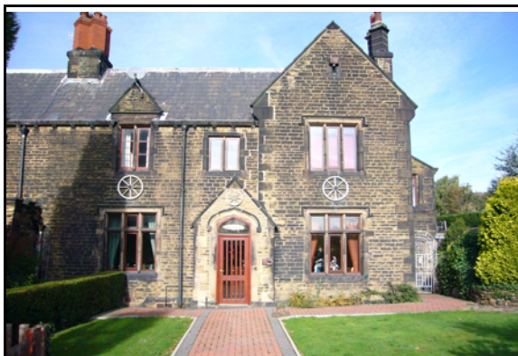
Replacement door and windows
