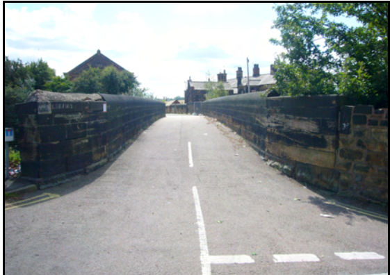
Railway Bridge to Cavendish Place
