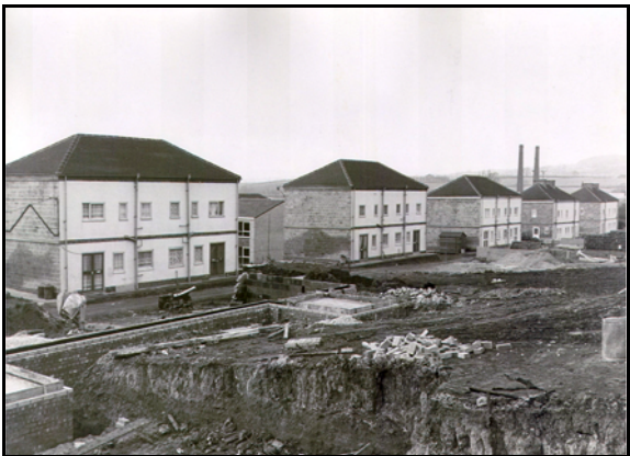
Workers houses with new blocks under construction 1975
