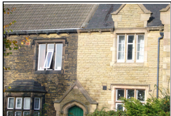
Replacement UPVc windows on the left
