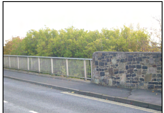
Replacement of stone boundary walls
