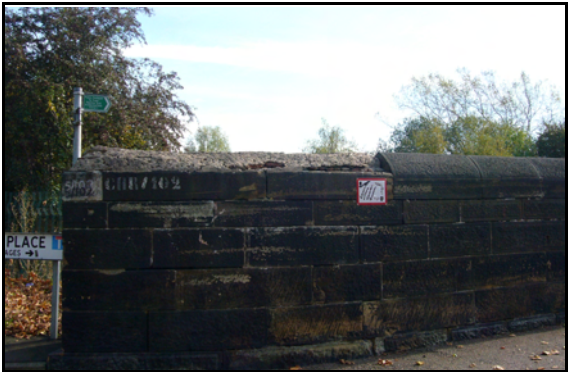
Concrete repairs to coping stone
