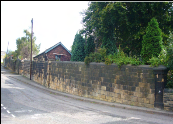
Stone wall to rear of Nos. 11-21 Station Road
