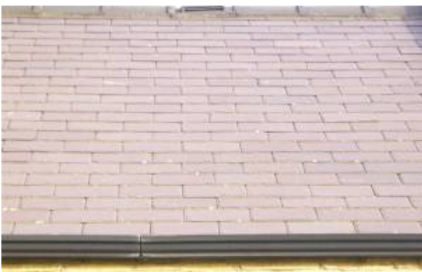
Slate roof on the Church
