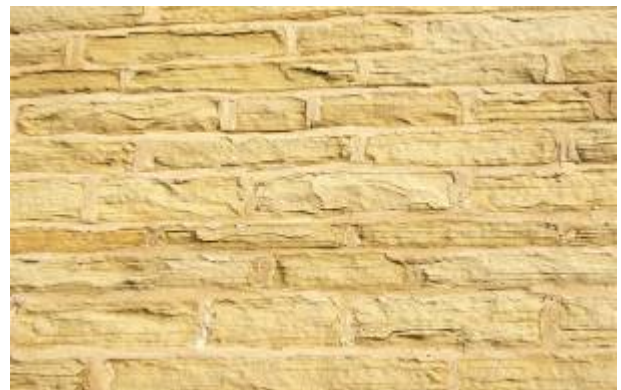
Coal measures sandstone wall
