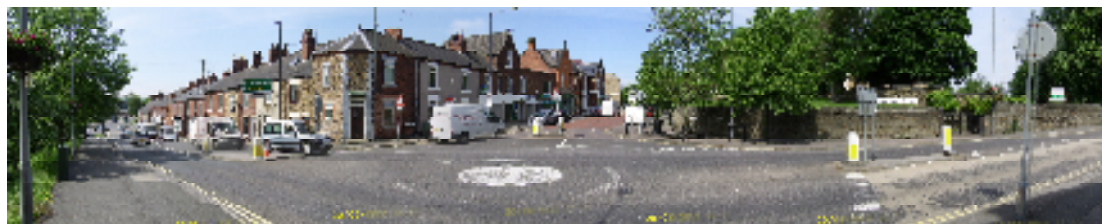
Figure 4.4.3 Northern Section of Façade and Carriageway
