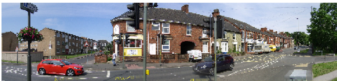
Figure 4.4.2 Affected Façade at Duke Street, Staveley
