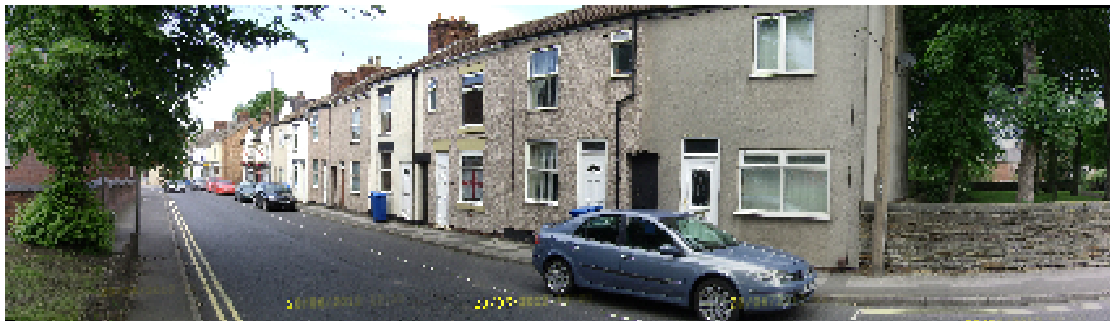
Figure 4.3.2 Affected Façade at Church Street, Brimington
