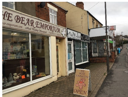
Figure 9.66: Bridge Street, Killamarsh
