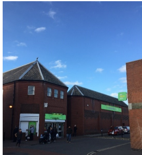
Figure 9.12: Co-operative Foods Supermarket, Victoria Street, Shirebrook
