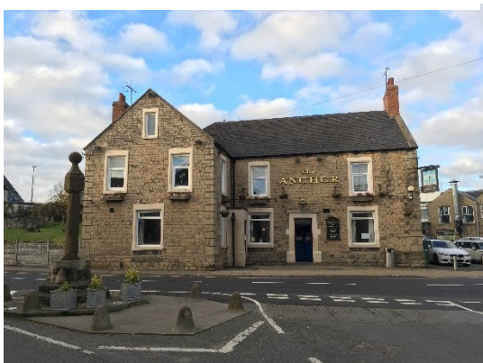
Figure 9.22: The Anchor Public House
