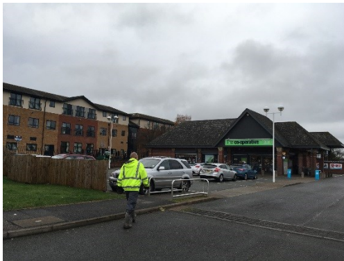
Figure 9.25: Co-operative Foods Supermarket, South Normanton
