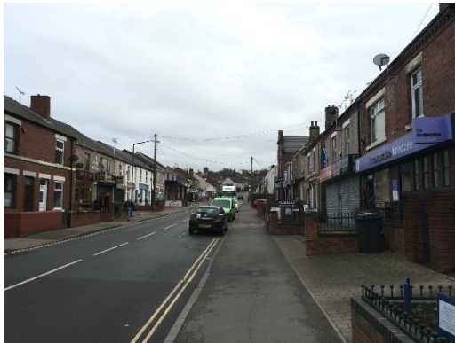
Figure 9.63: Northern Bridge Street, Killamarsh
