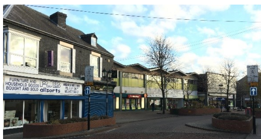
Figure 9.45: High Street, Staveley (looking south)
