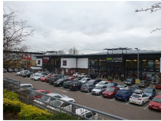
Figure 9.37: Ravenside Retail Park
