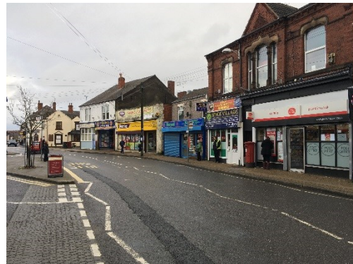
Figure 9.26: Market Place, South Normanton (looking south)
