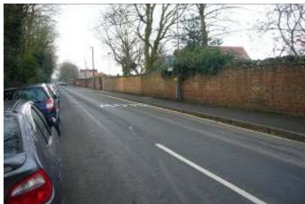
Walls on the south boundary
