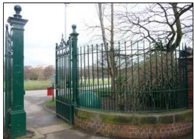
Pedestrian gate flanked with railings
