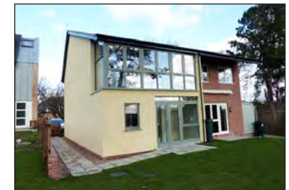
A large window for solar gain and a deep overhang and canopy for shade
