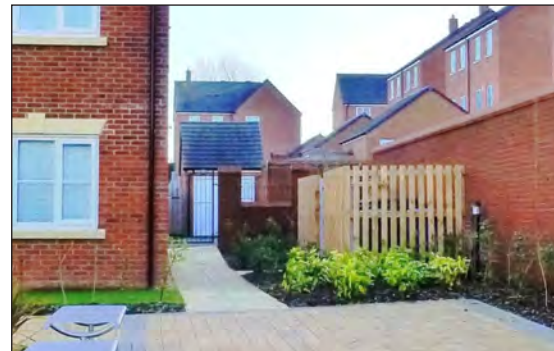
Above: Communal bin stores positioned discretely between buildings with a short level access to the street for ease of access on collection day
