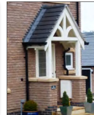
A meter box sited discretely within a porch enclosure
