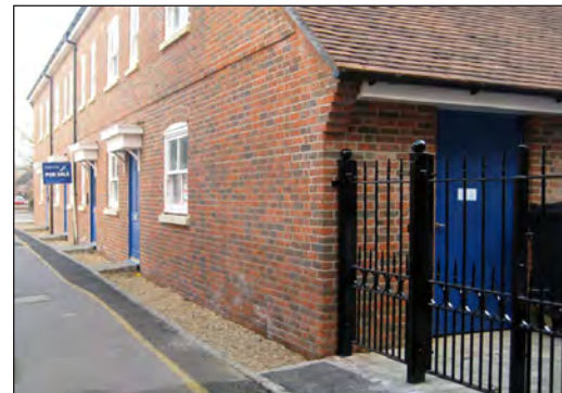
Above: Communal bin storage integrated into a lean-to, behind a secure gate and with external access only
