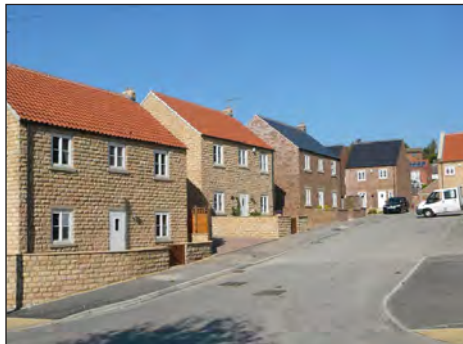
A central village development with a minimal set-back and robust boundary walls
