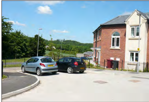
Cars parked within a turning head cause an obstruction to service vehicles needing to turn
