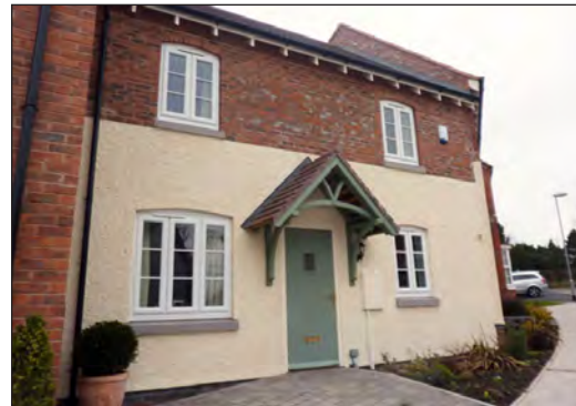
An attractive quality canopy and door relate to the street while a level threshold affords access for all
