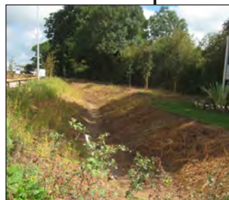
SUDS swales in a green corridor
