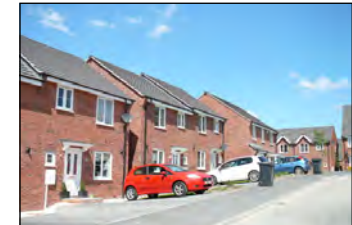
Parking occupying whole frontages dominates the street scene and detracts from its appearance.
