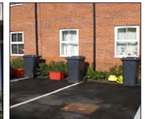
Above: Bins obstruct parking where insufficient space has been provided to store waste and recycling containers
