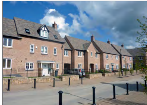
A continuous building line clearly defines the frontage
