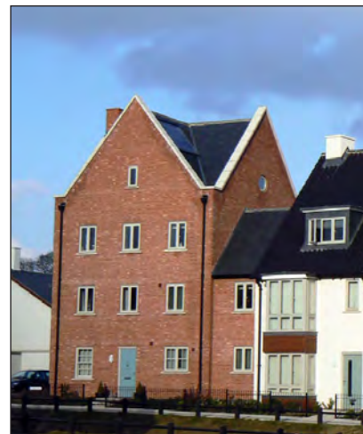
A notable corner expressed through scale, height and roof form of the house
