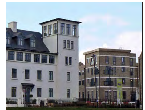
Corners emphasised by height and architecture identify an important node and aid legibility
