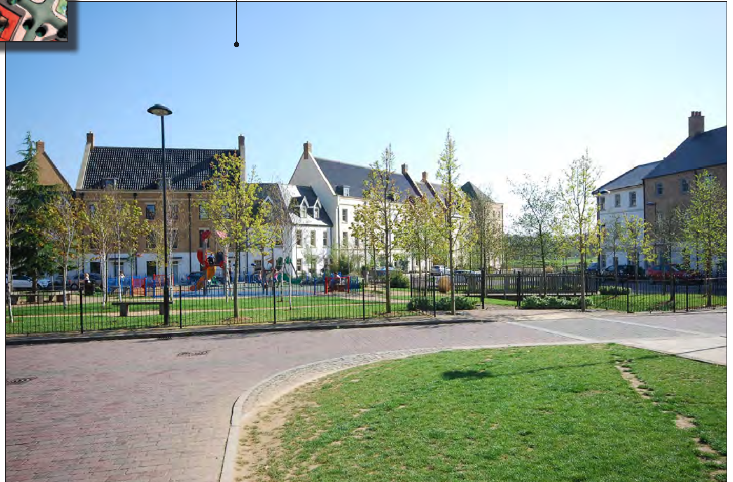
Permission to use drawing and photo courtesy of the Homes and Communities Agency
