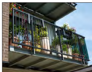
Centre and right: Balconies to individual flats provide a modest private space that allows scope for personalisation
