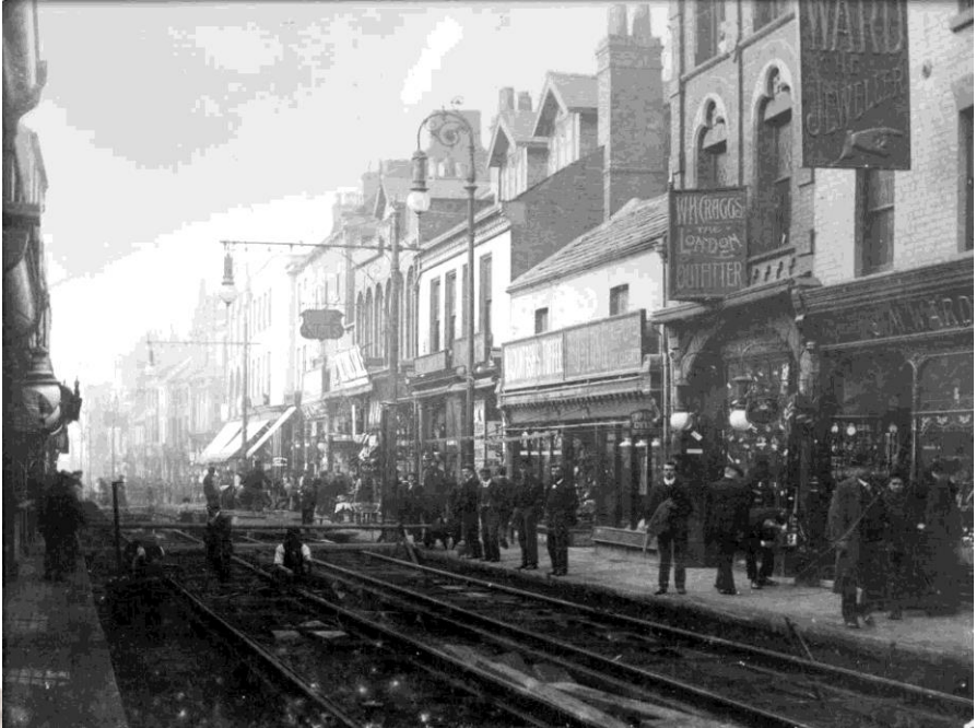
Laying electric tramlines along Burlington Street and High Street, Chesterfield, 1904.
