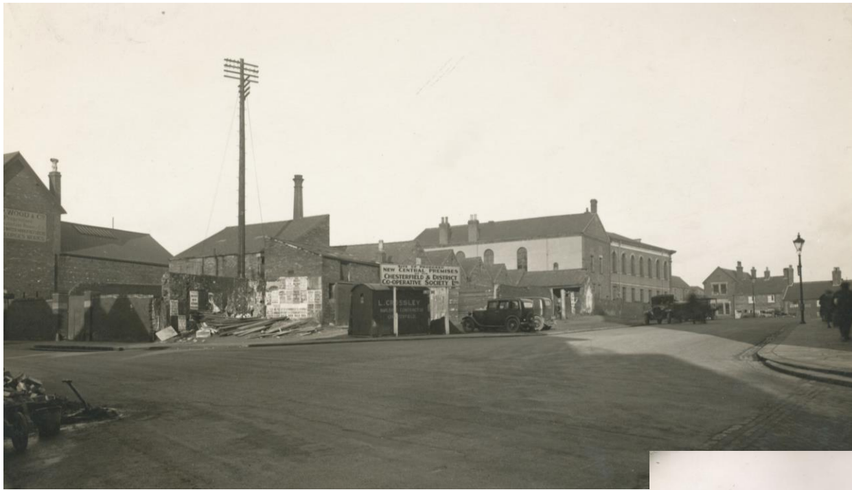
The new site, on the corner of Elder Street, for the soon to be built Chesterfield & District Co-op.
