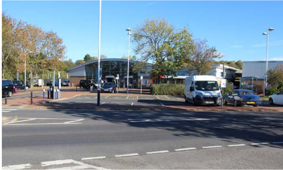
Existing view of the station facing the forecourt
