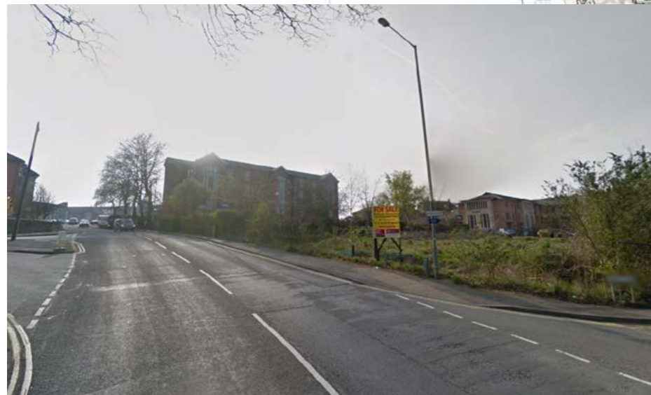
Existing view along Brewery Street
