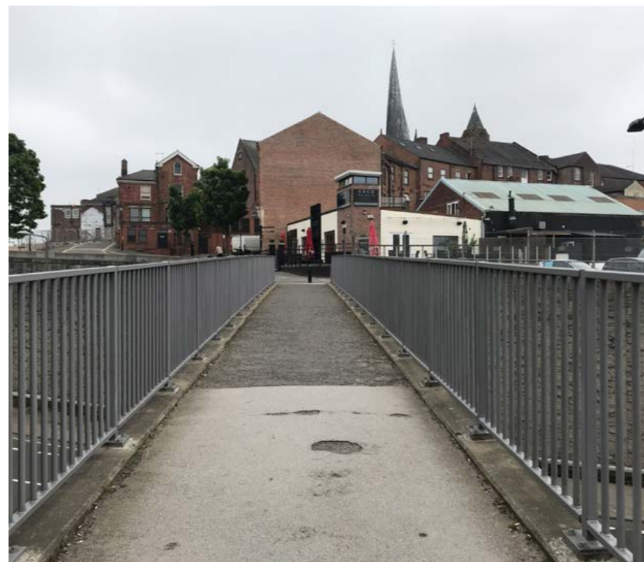
3. View toward Corporation Street from current pedestrian bridge
