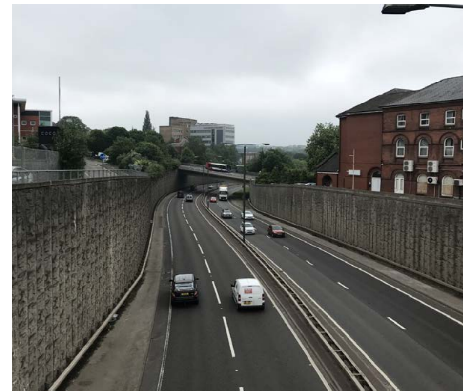
10. View north along the dual carriageway
