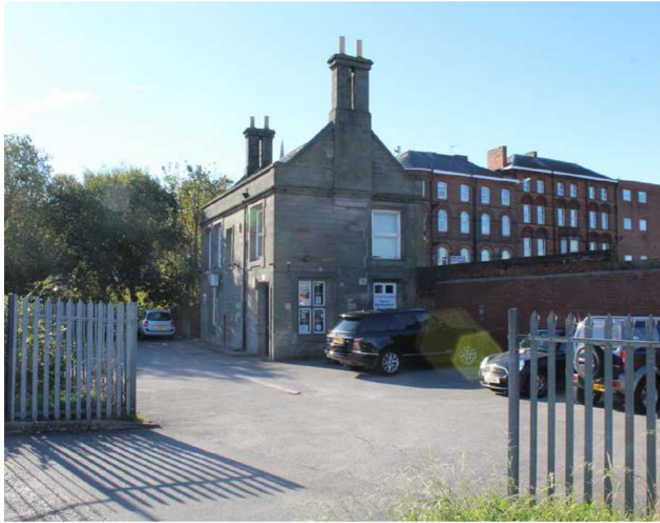
Grade II Listed Engineers Office (Study Area)
