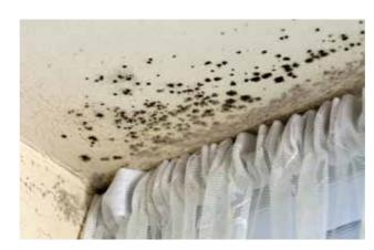
Tenants sometimes contact us because they believe they have damp in their home but mostly the problems are caused by condensation. Condensation is caused by people failing to ventilate the property and not as a result of any property defect.
