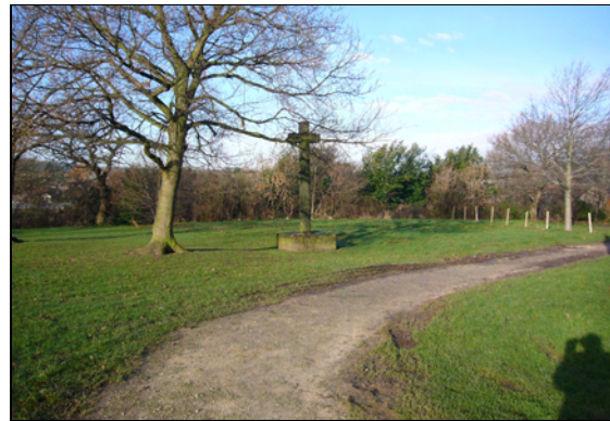
Footpath to the Chapel destroyed by cars
