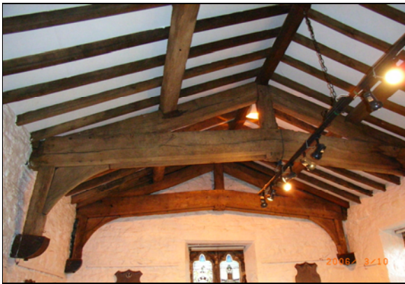
Internal roof structure
